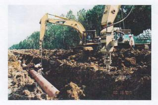
For those areas not conducive to auger anchors BKW offers the slot weight. The slot weight is made of tough polyurethane and supported by nylon straps for strength. The slot weight weighs 100 lbs. and uses the backfill for weight: this lowers the cost of hold down by 50% over concrete set-on weights or sacks.
